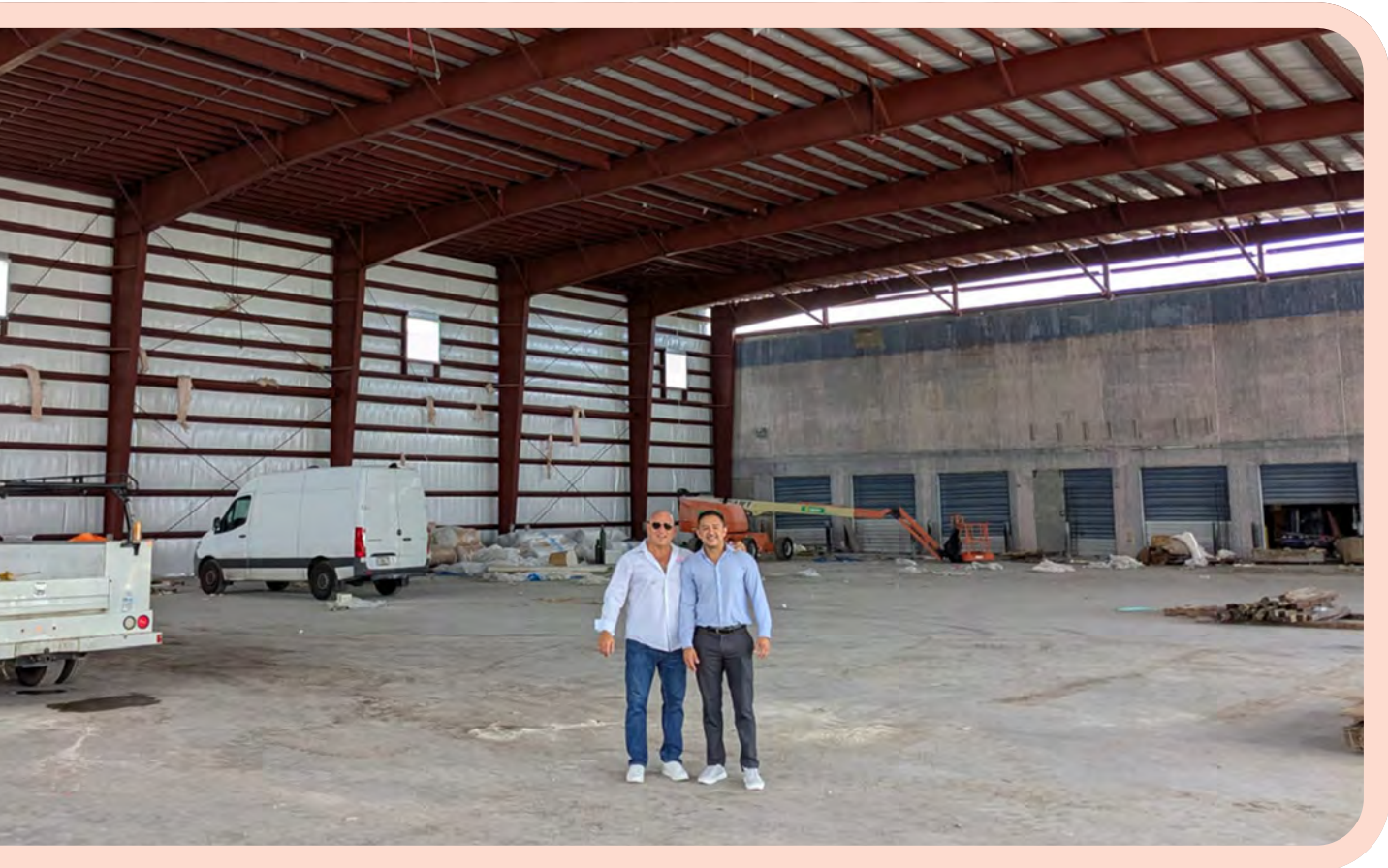
Family business: the expansion of the company’s building by 30,000sq ft will allow for two additional converting lines
