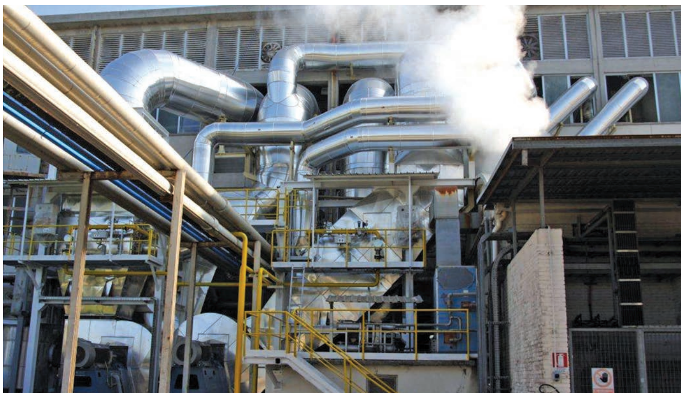
Moving the air system outside has reduced the fire risk
