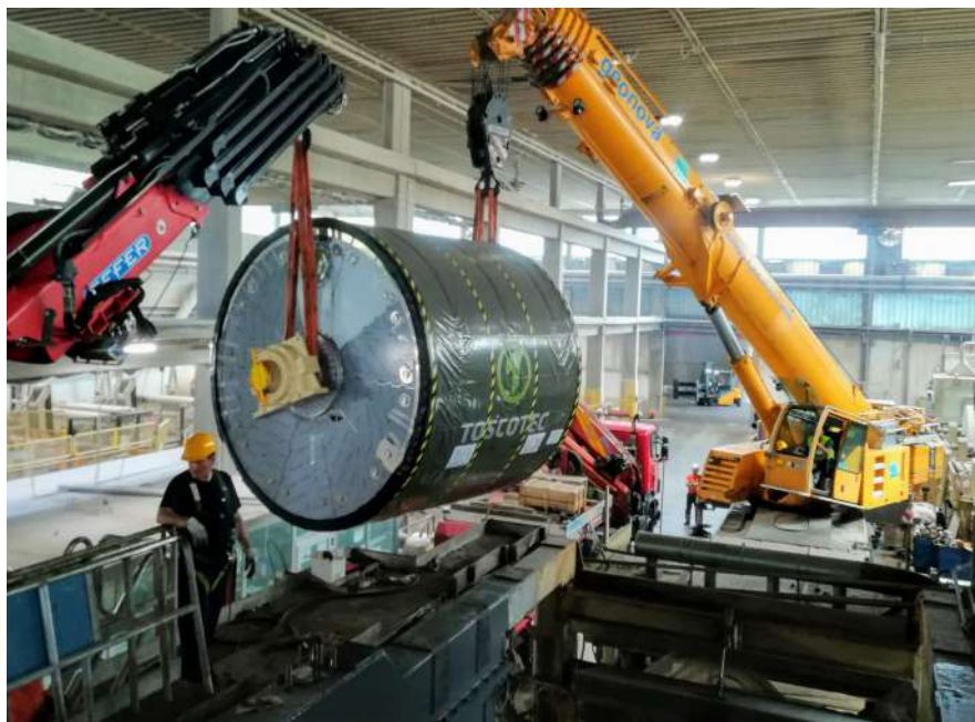
Capacity boost: Work on replacing existing Yankees with Toscotec's second-generation Steel Yankee Dryers at Lucart's Diecimo tissue mill
